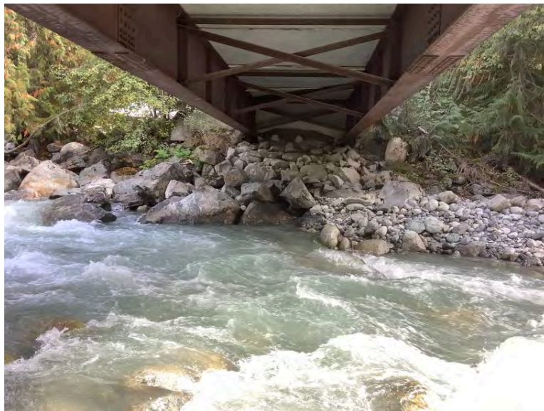
Left Bank Abutment when facing downstream
