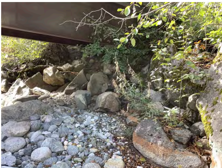
Right Bank Abutment when facing downstream
