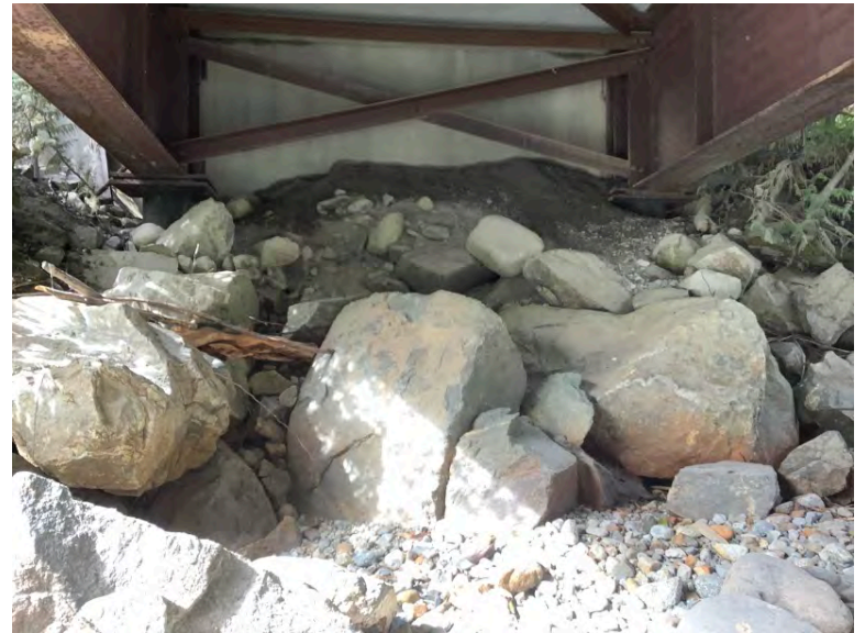
Right Bank Abutment when facing downstream
